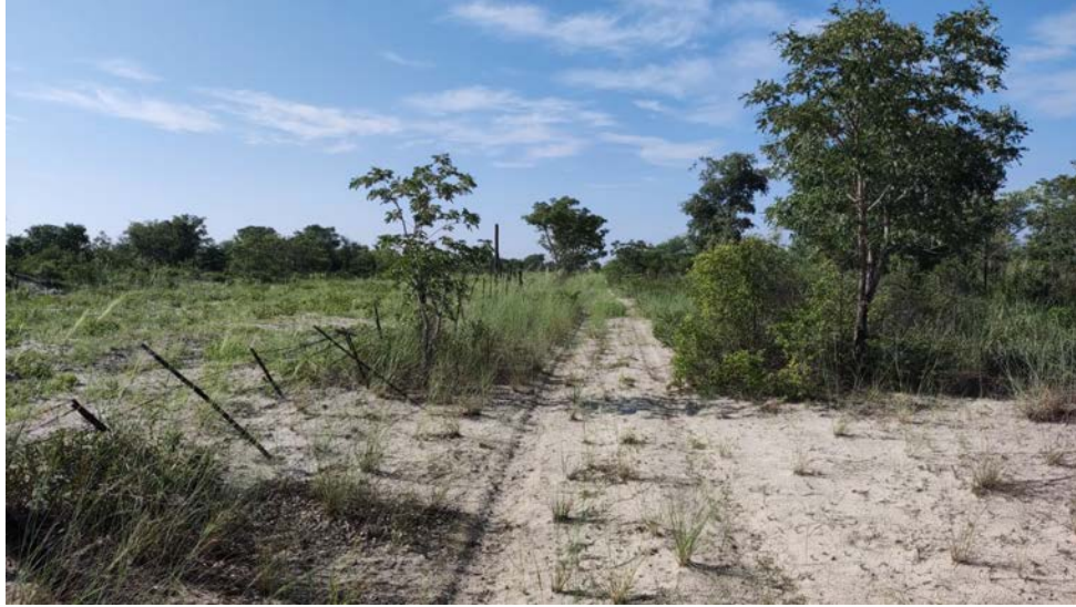
Figure 23. Partly down fence adjacent to Khaudum National Park. Photo: Markus Hofmeyr.
