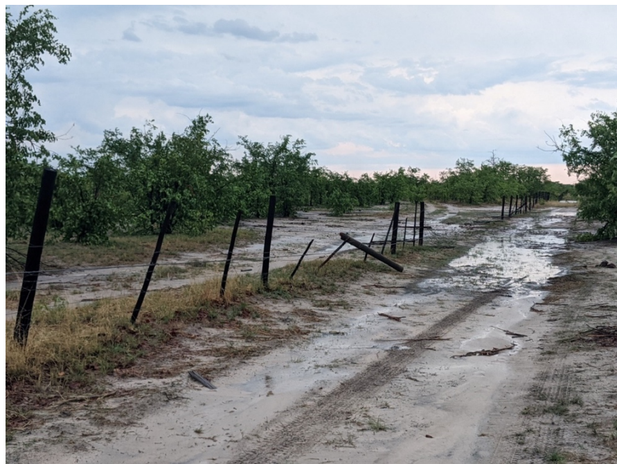
Figure 18. Northern Buffalo fence in poor condition with missing wires and major breaks during a site visit in November 2022.
