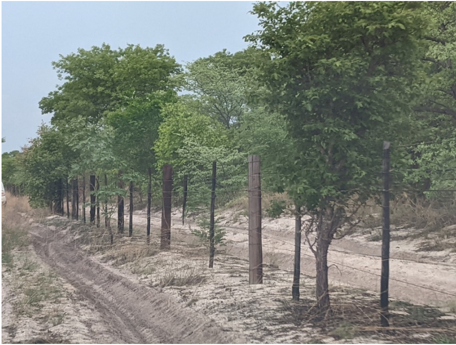
Figure 17. Northern Buffalo fence in good condition, although with a lack of bush-clearing, as observed during a site visit in November 2022.
